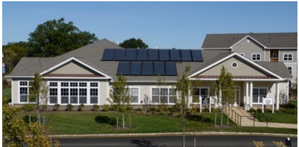
Avalon West Long Branch (NJ): Solar panels installed on community clubhouse.
